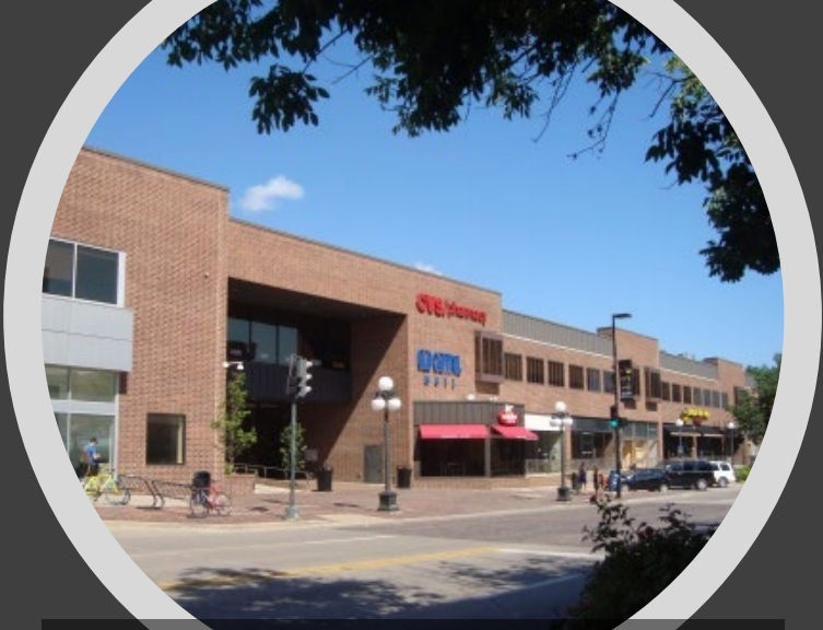
University Capitol Centre – Remodel Space for Chief Diversity Office and UI Service Center $3.3 Million
